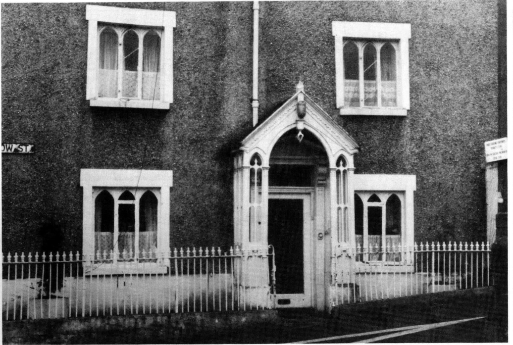
Fig. 5a The Willows, Llangollen, Clwyd. Original doorcase within a later porch
